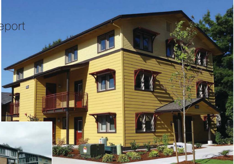
Stellar Apartments in Eugene, Ore., consists of two nearly identical low-income apartment buildings built to different sustainable standards. One meets the city's Earth Advantage Program requirements, while the other (pictured above and left) is the first multifamily building to achieve Passive House certification. The Building Team included St. Vincent DePaul Society of Lane County (owner), Bergsund DeLaney Architecture & Planning, Hohbach-Lewin Inc., Poage Engineering, and Dougherty Landscape Architects.
